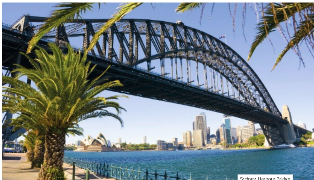
Sydney, Harbour Bridge
